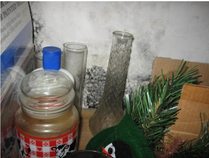
Mold on drywall under basement bathroom sink.
