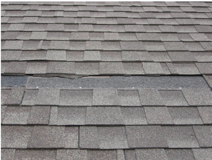
Missing shingle on roof that needs to be replaced.
