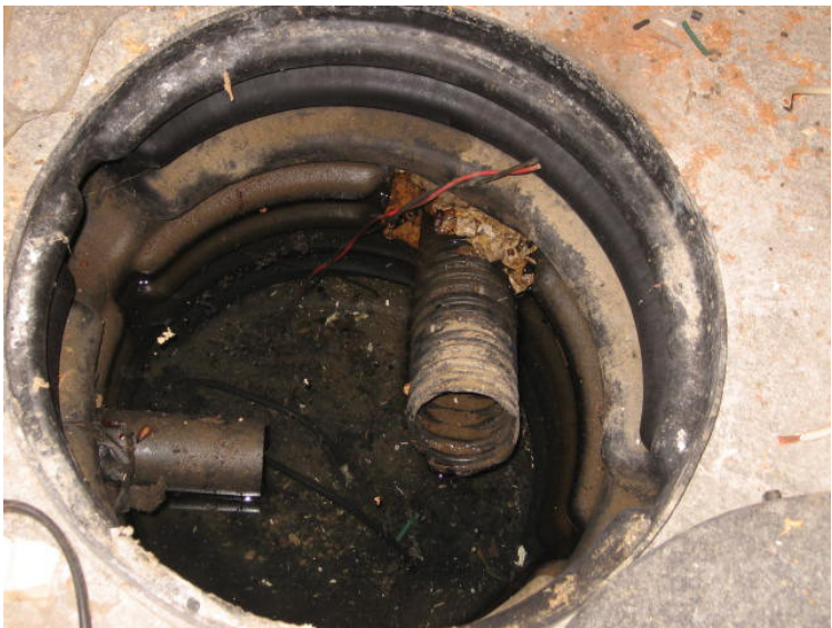
No sump pump installed in pit in basement.
