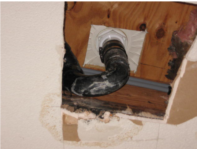
Master bathroom shower leaking into garage.
