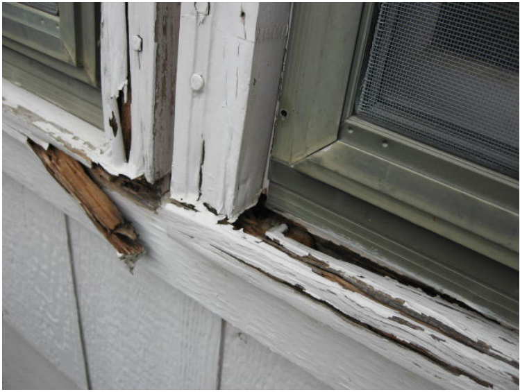
Rotted window trim that needs to be replaced.
