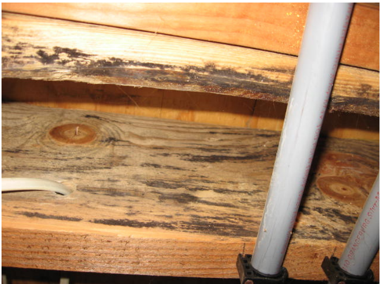
Mold on floor joists in basement.
