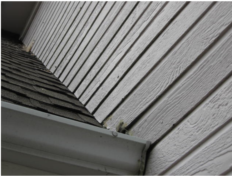
Siding buckled and too close to shingles.
