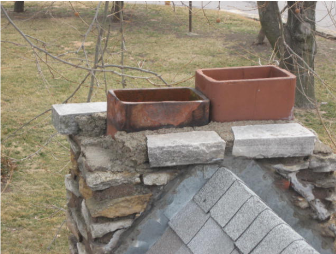
Damaged crown on fireplace and no flue caps.
