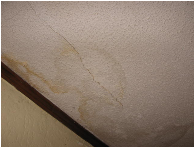
Water damage on ceiling in dining room.
