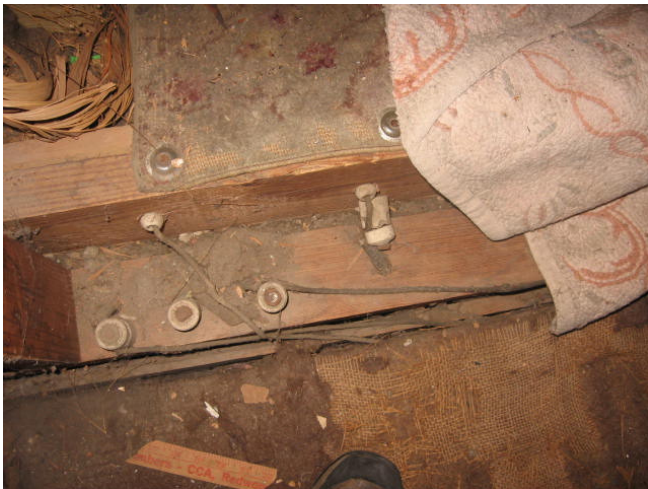
Knob and tube wiring in attic.
