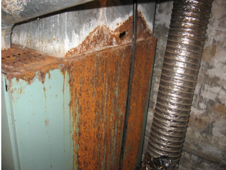
Rust on hot water heater.
