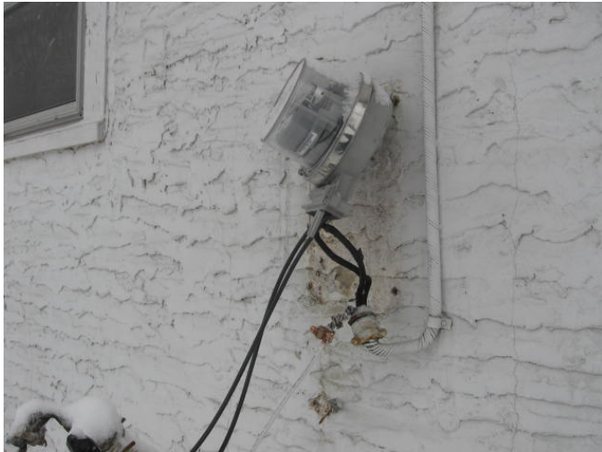
60-amp box not secured to house.
