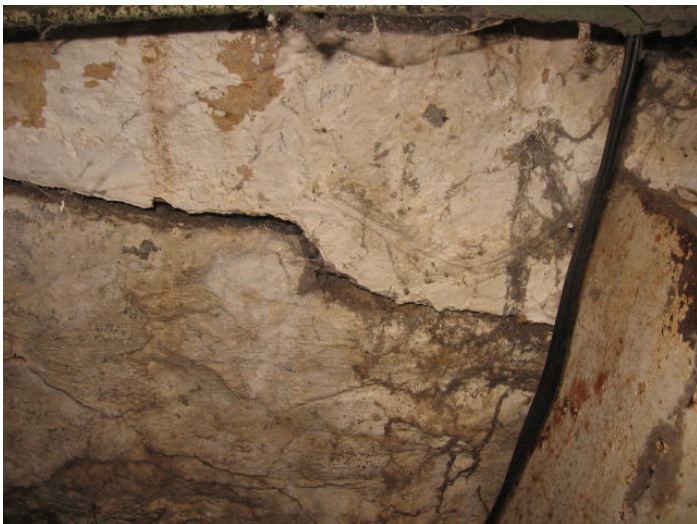
Crack on foundation wall.
