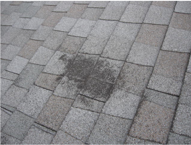
Damaged shingles on roof.
