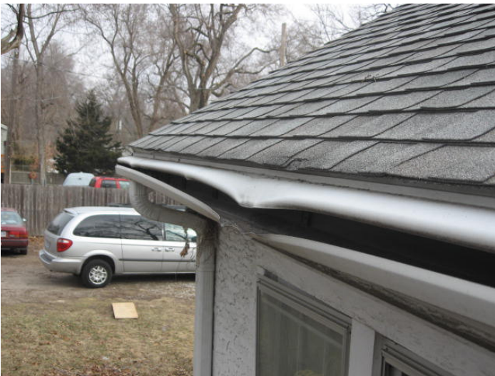
Damaged gutter.
